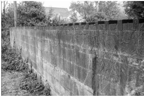
Figure 3. A masonry portion of the Hall's Hill segregation wall - date unknown (Image courtesy of Columbia University).
